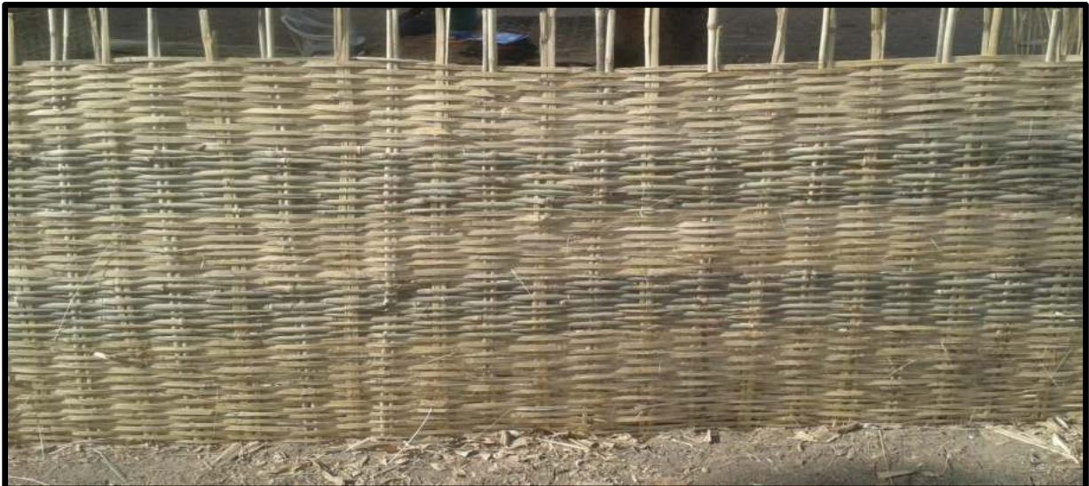
Photo : palissade (crinting)
